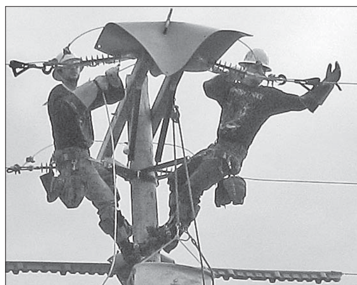
ABOVE AND BELOW: Modesto Irrigation District team competes in the double dead end 4 poly bell change out.
