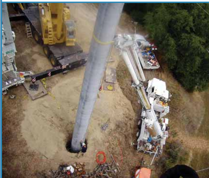
A pole is positioned in a deep hole, where it will be anchored with plenty of concrete.
