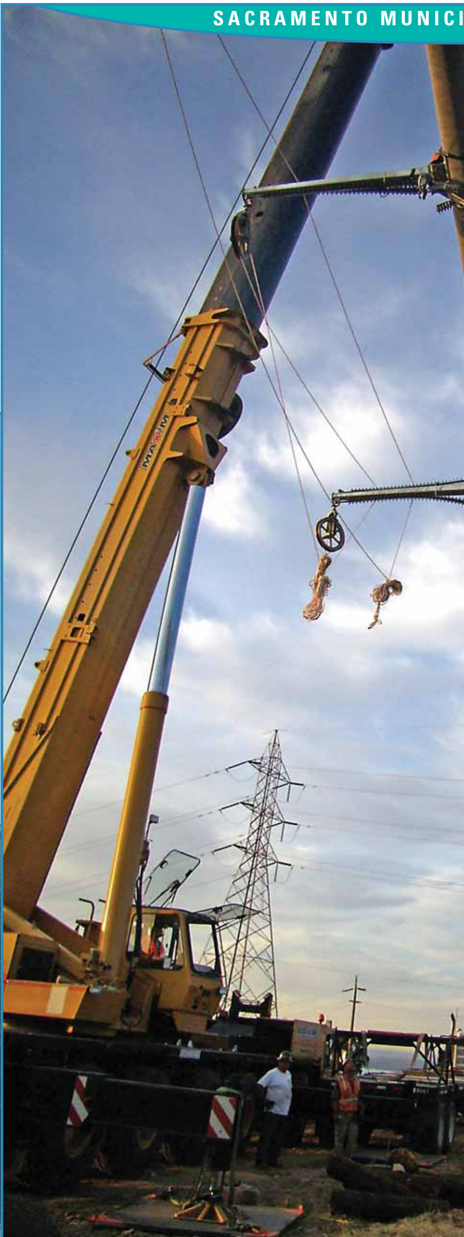
SMUD crew (above) installs a steel transmission pole in two pieces. Poles weighing between 40 and 70 thousand pounds are hefted into position (below and right).
