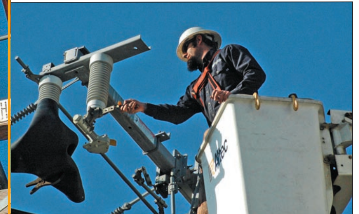
Ty Wyatt installs a switch terminal that will connect to the newly-replaced underground system.
