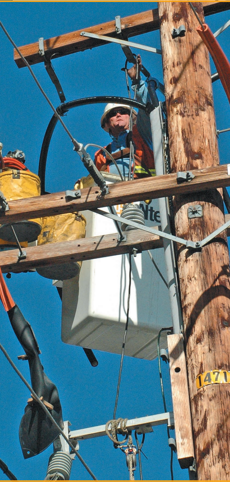
Skip Alcorn relocates a temporary protective grounding cable in order to land the new 1100 Al cable at top of riser pole.
