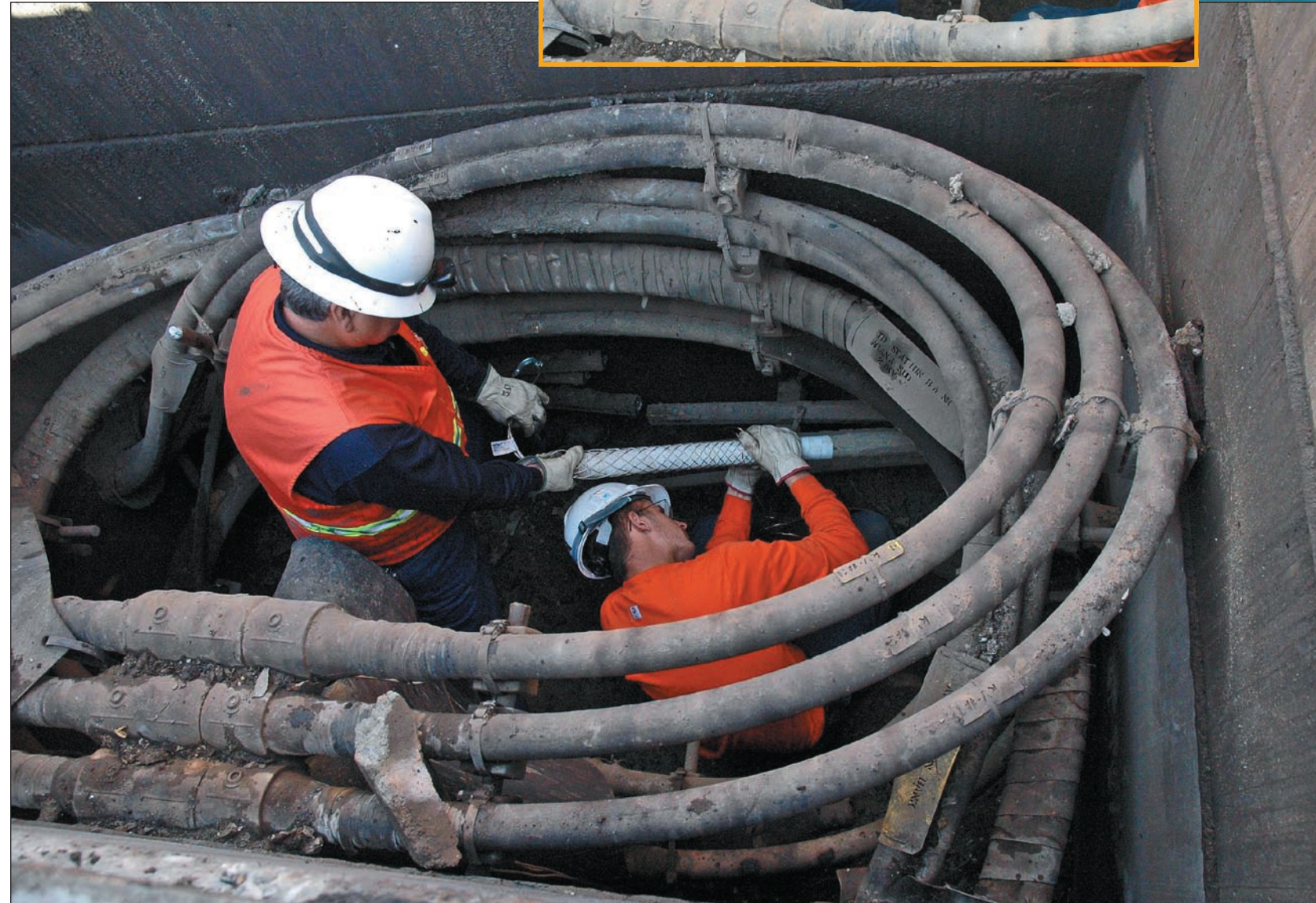
Mike Farinsky, Jr. secures a Kellum grip on to a cable in order to pull in braided rope on Soquel Avenue in Santa Cruz. Working in the vault with him is J.D. Sotelo.
