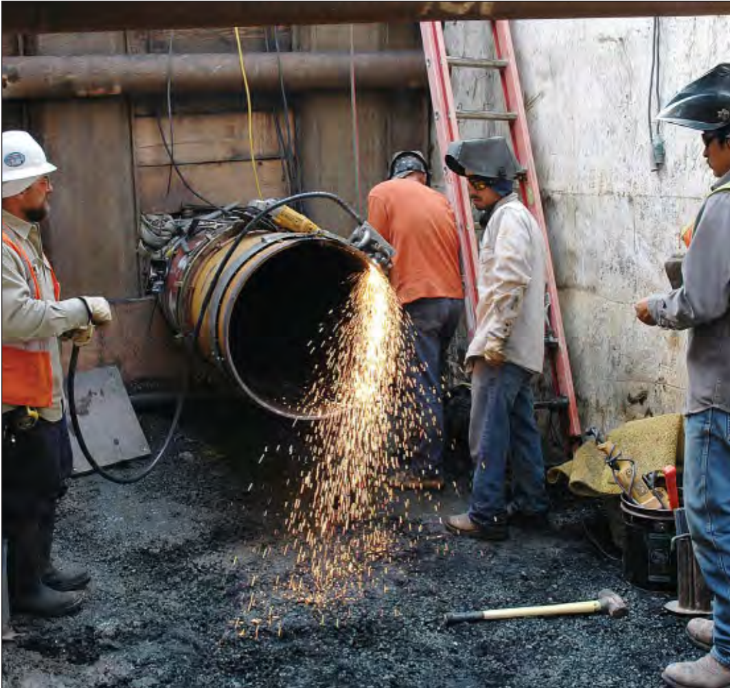
Sparks fly as the pipe is beveled.
