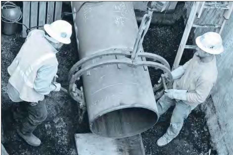
T.C. Gotcher, left, and Eric Tague position the pipe clamp.
