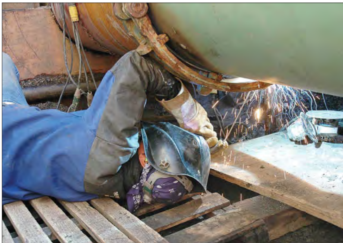
Making the weld on the inside of the pipe.
