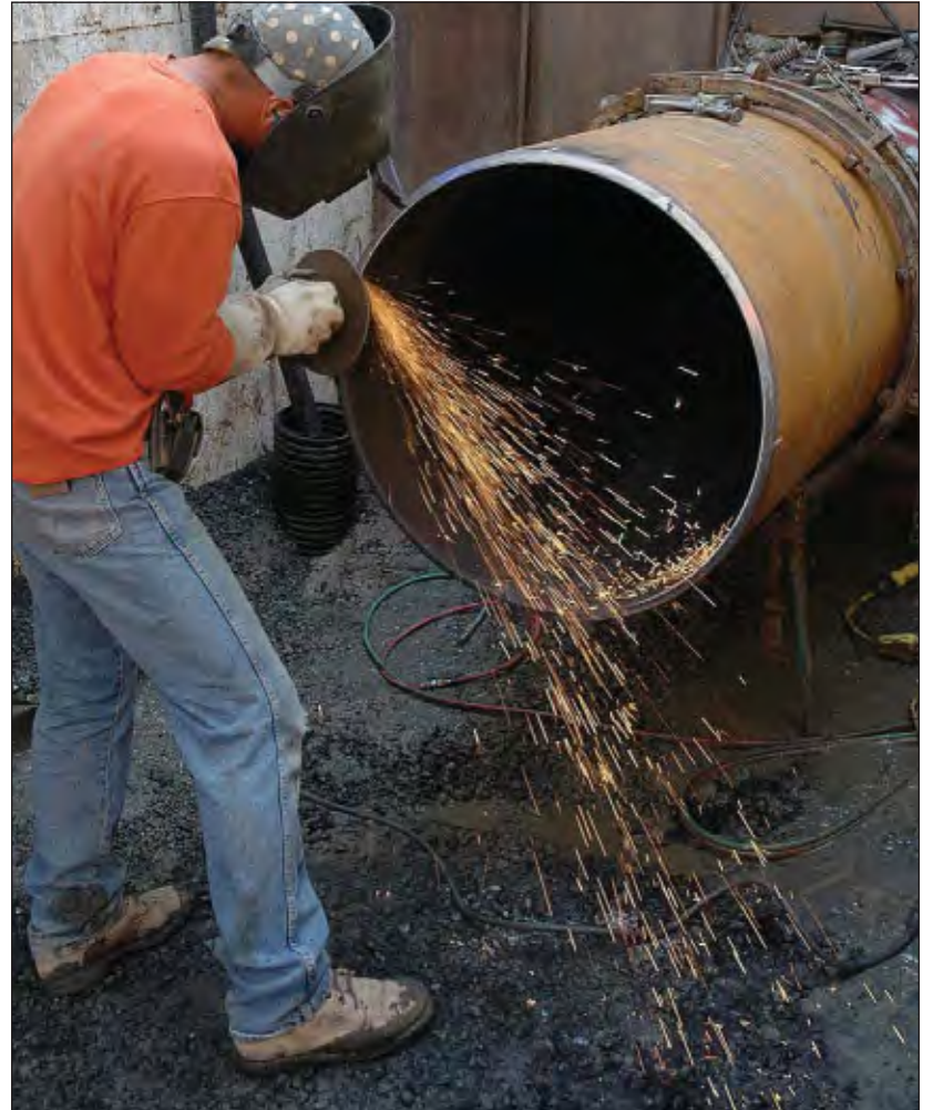
Prepping the pipe ends to weld.
