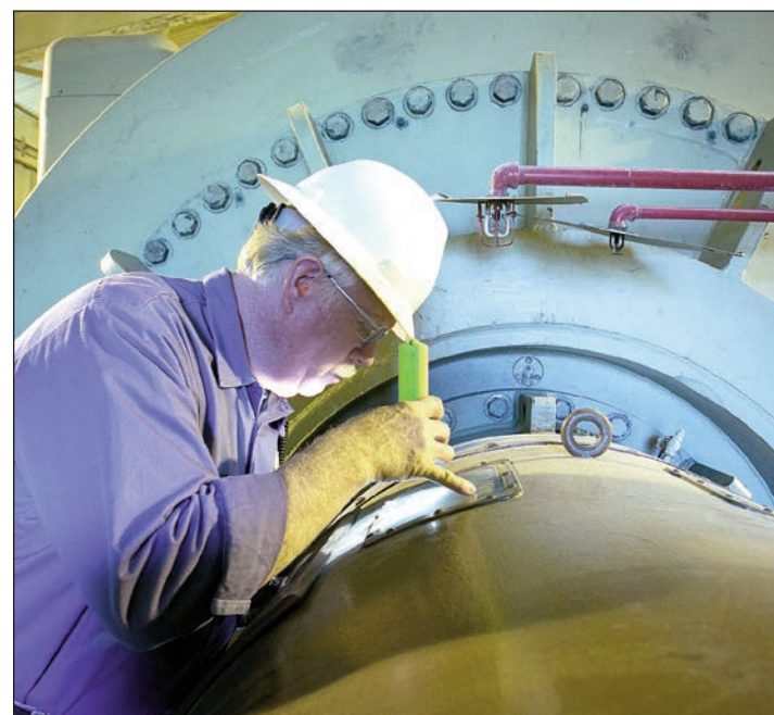
Gary Detrick, in the unit #2 turbin house, inspects the brushes on the collector end of the turbin.
