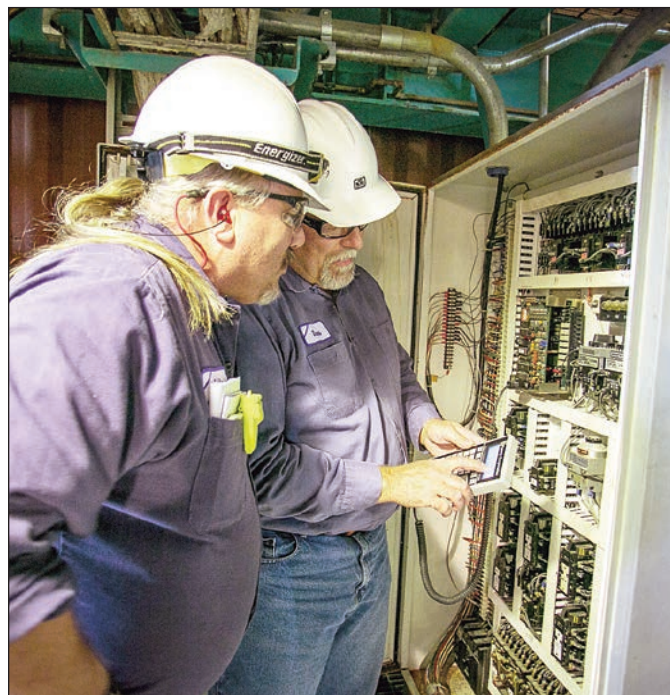
Right: Duane Matheus and Eddie Eubanks troubleshoot the #1 gas burner on the unit #1 boiler "A" deck firing aisle.
