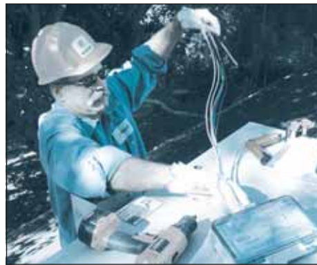
Bob Karle reconnects a radio-controlled cyclor on the air conditioner of one of SMUD's participating customers.
