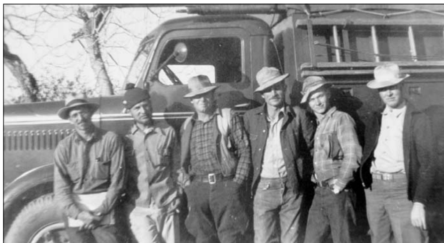
The union was still trying to get a foothold at PG&E when this photo was taken of a Placerville crew with a new 4-wheel drive truck in 1947. From left are Ralph Silva, foreman; Bill Smith, groundman; Robert Glasgow, lineman; Fred Yoeman, groundman; George Besse, groundman; Lonnie Evans, truck driver. IBEW 1245 Archive
