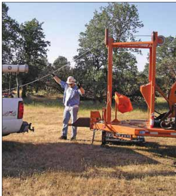
Lineman Brian Adams preparing to start fiber pull.
