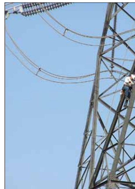
Apprentice Lineman James Clark climbs 50
