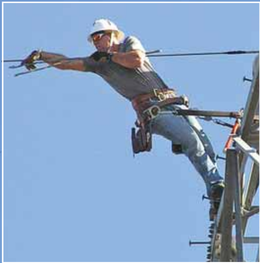
Apprentice Chad Rocco stretches out in his belt to remove a preform from the existing static.
