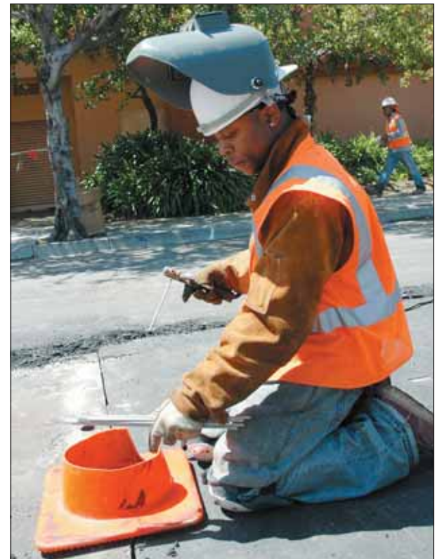
Marquez Boyd, one of the job fair recruits, is about to finish up some welding.
