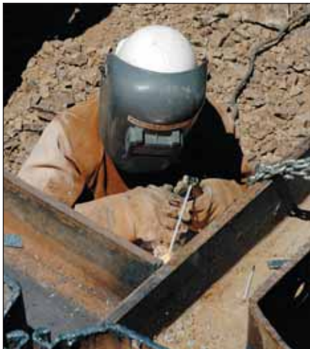
Welding part of the shoring system for a manhole.
