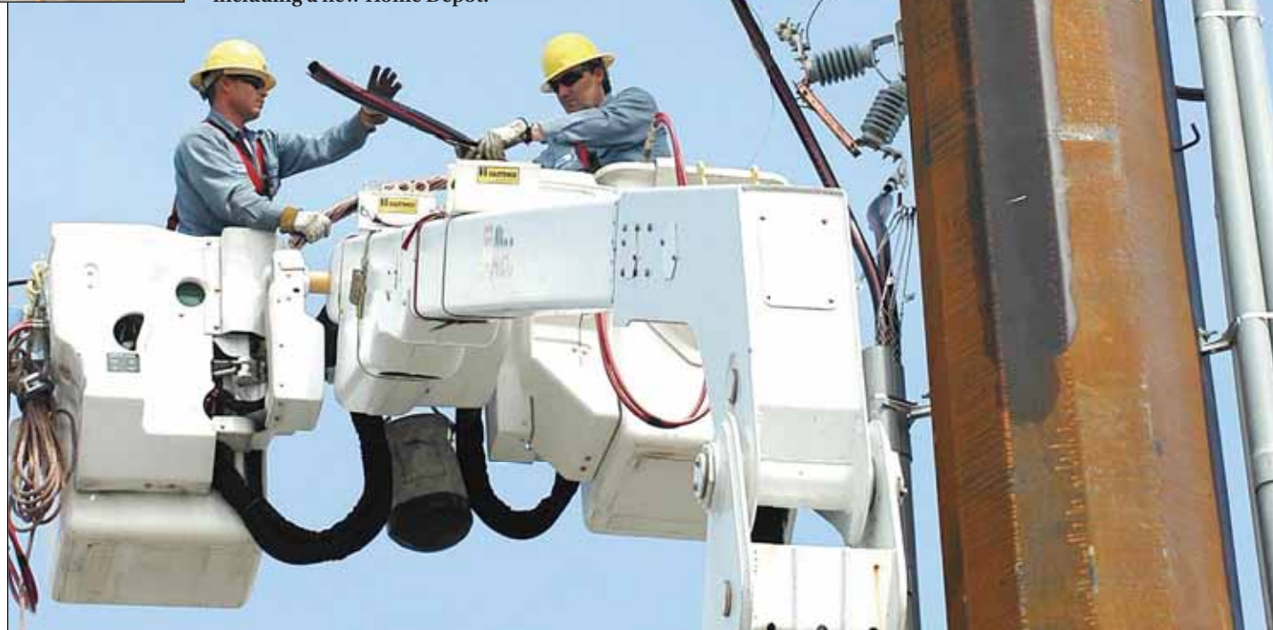
Casey Guinn, left, and Troy Borges work on the installation of three new feeders to the substation at Hatch and Central in Turlock. A lot of load has been added on this road recently, including a new Home Depot.
