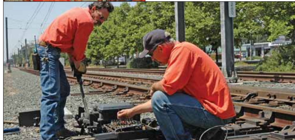
BELOW: Johnson and McCord perform preventative maintenance on a rail switch.
