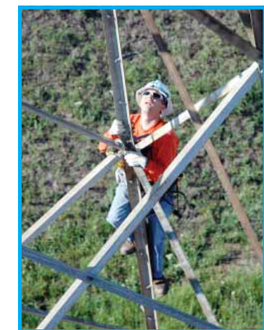
Travis Bess maintains 3-point contact on his way up the tower.
