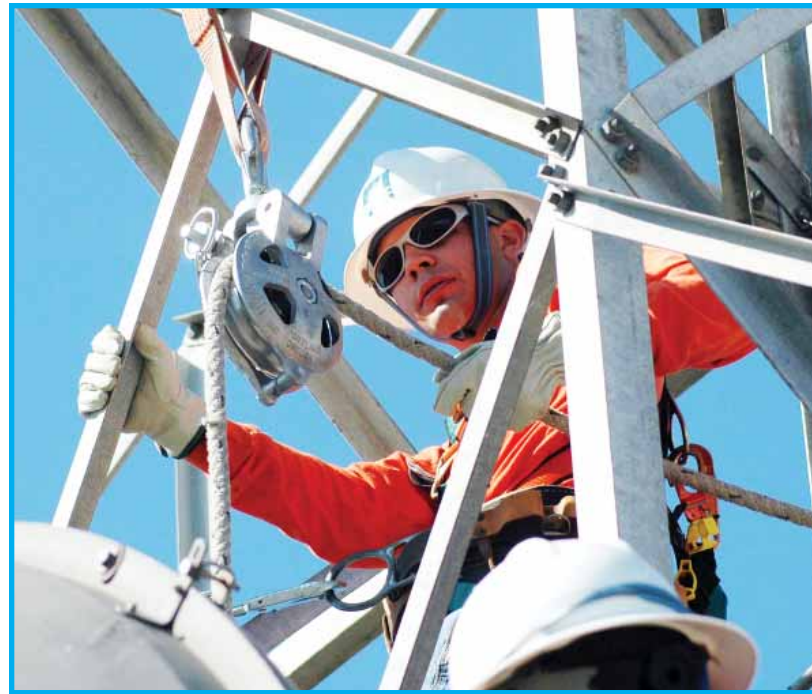
Travis Bess has just finished setting the load line for the dish removal.
