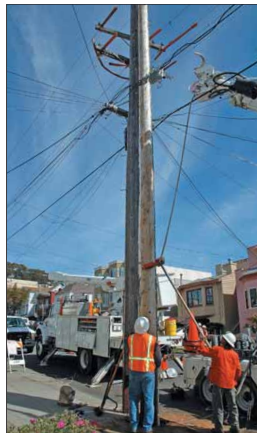
Marshall Free removing rigging after setting the pole.
