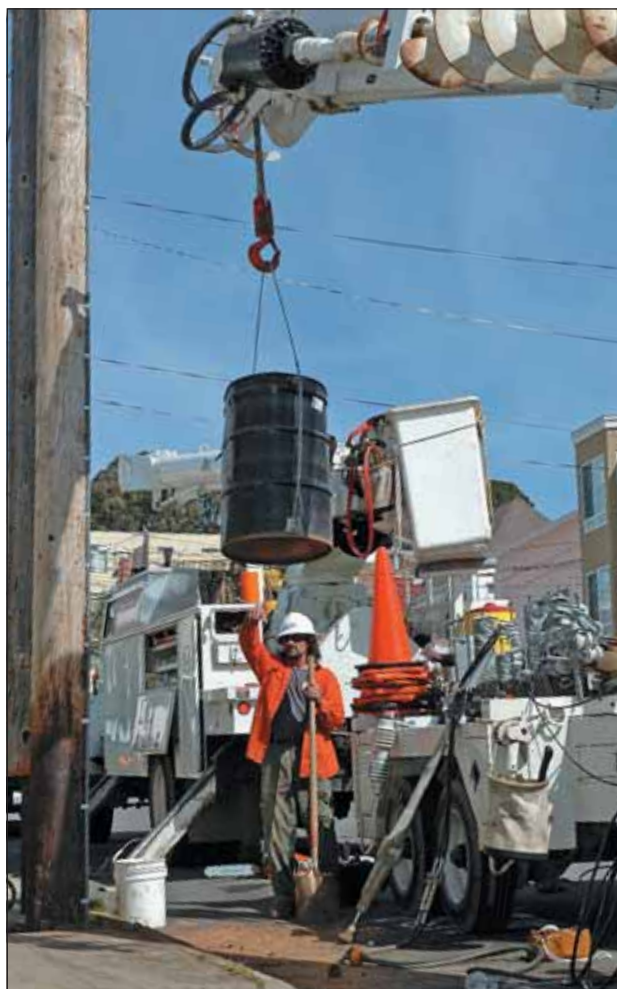
(RIGHT) Marshall Free guides a bucket of fill into position.
