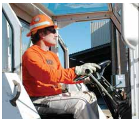
Apprentice Lineman Mark Regan operates the crane.
