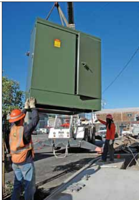
Apprentice Lineman Michael Hamill, left, and Lineman Al Fortier guide the 10,000-pound transformer to the pad. Operating the crane is Apprentice Lineman Mark Regan.
