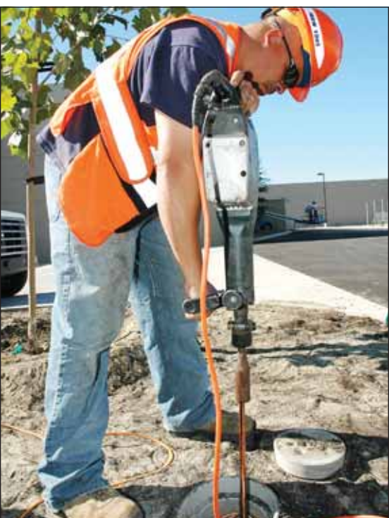
Groundman Eddie Courtney secures the transformer to the pad.
