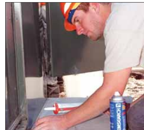
Groundman Michael Stover applies caulk to the transformer.
