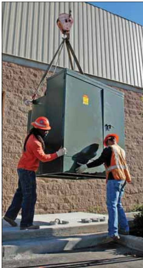
Apprentice Lineman Michael Hamill, left, and Lineman Al Fortier guide the 10,000-pound transformer to the pad. Operating the crane is Apprentice Lineman Mark Regan.
